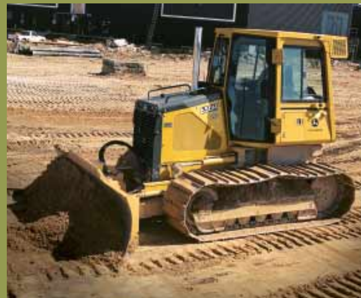
At left, most earthmoving consisted of truck loading at the $46-million Baltimore-Washington International (BWI) Airport project. Above, a 650H Dozer prepares the grade for utility installation. Flanigan's BWI managers above are Steven Wellen, left, project superintendent, and Keith Jones, project manager.
